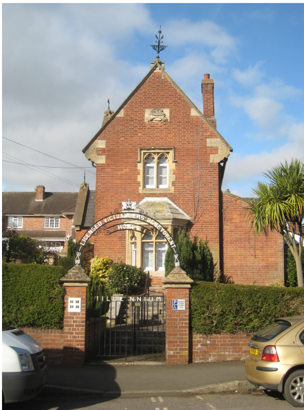
Elevation from street
